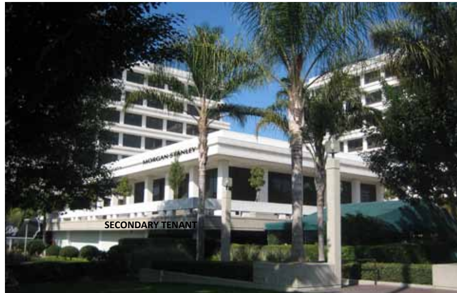
ST 6.6 - VIEW FROM NEWPORT CENTER DRIVE - BUILDING 860/880
