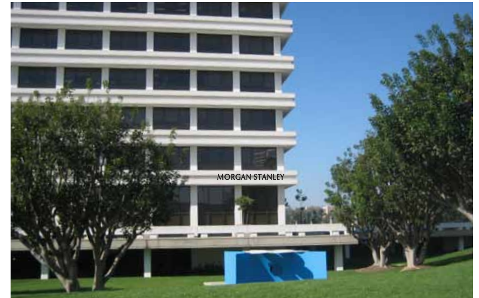
ST 6.8 - VIEW FROM NEWPORT CENTER DRIVE - BUILDING 800
