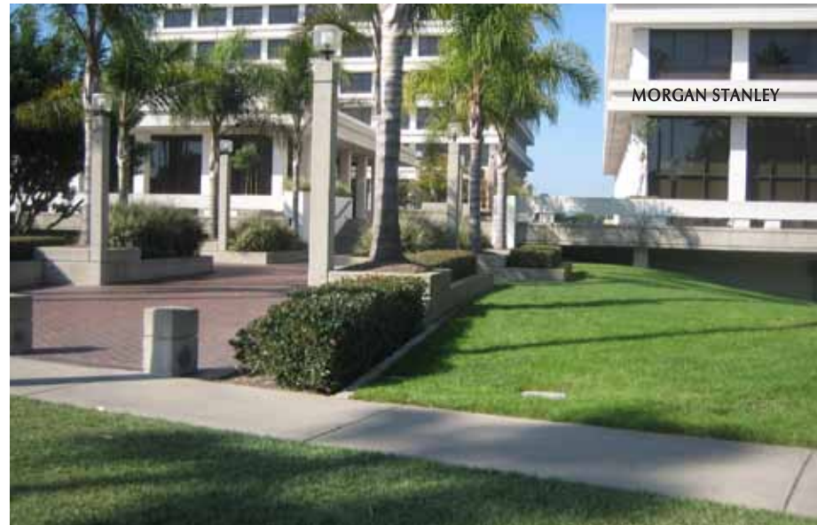
ST 6.7 - VIEW FROM NEWPORT CENTER DRIVE - BUILDING 800
