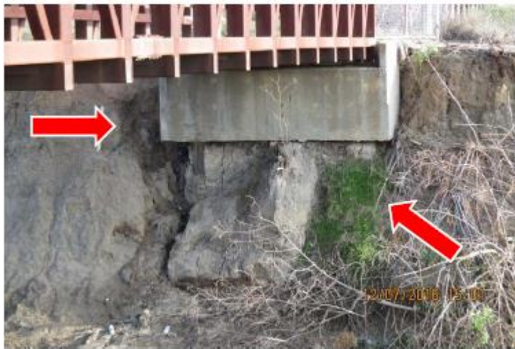
South Abutment, December 2016
