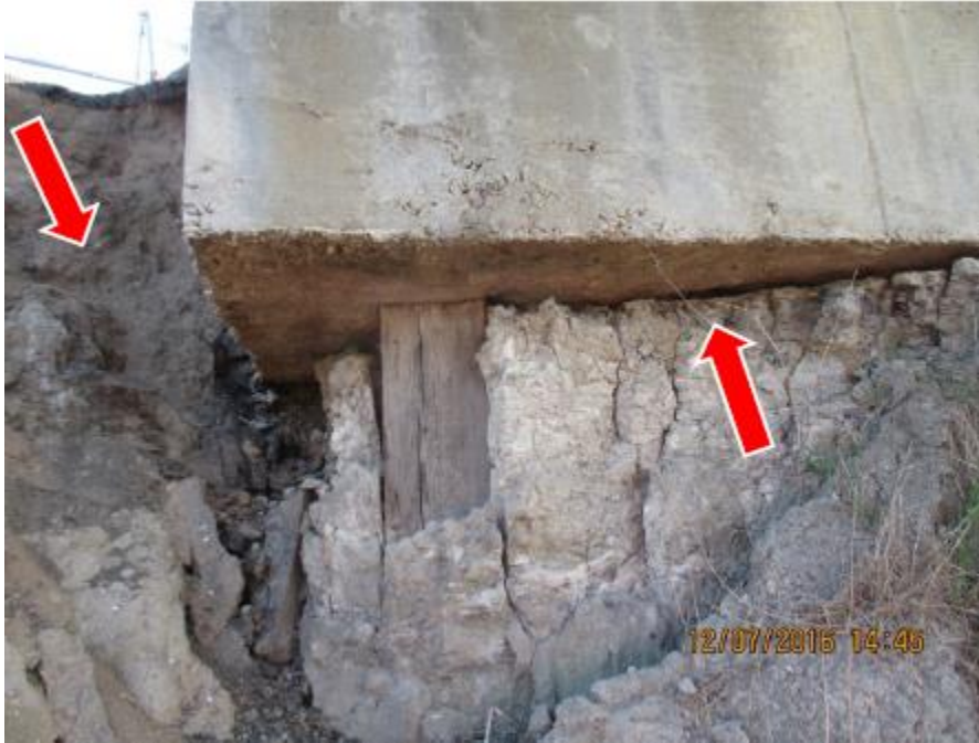
Exposed east pile at South Abutment
