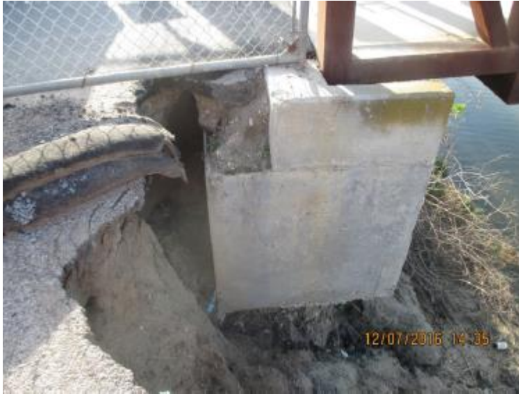
South Abutment, December 2016
