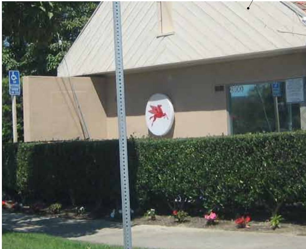
1 EXISTING CONDITION - MOBIL ON-BUILDING SYMBOL
