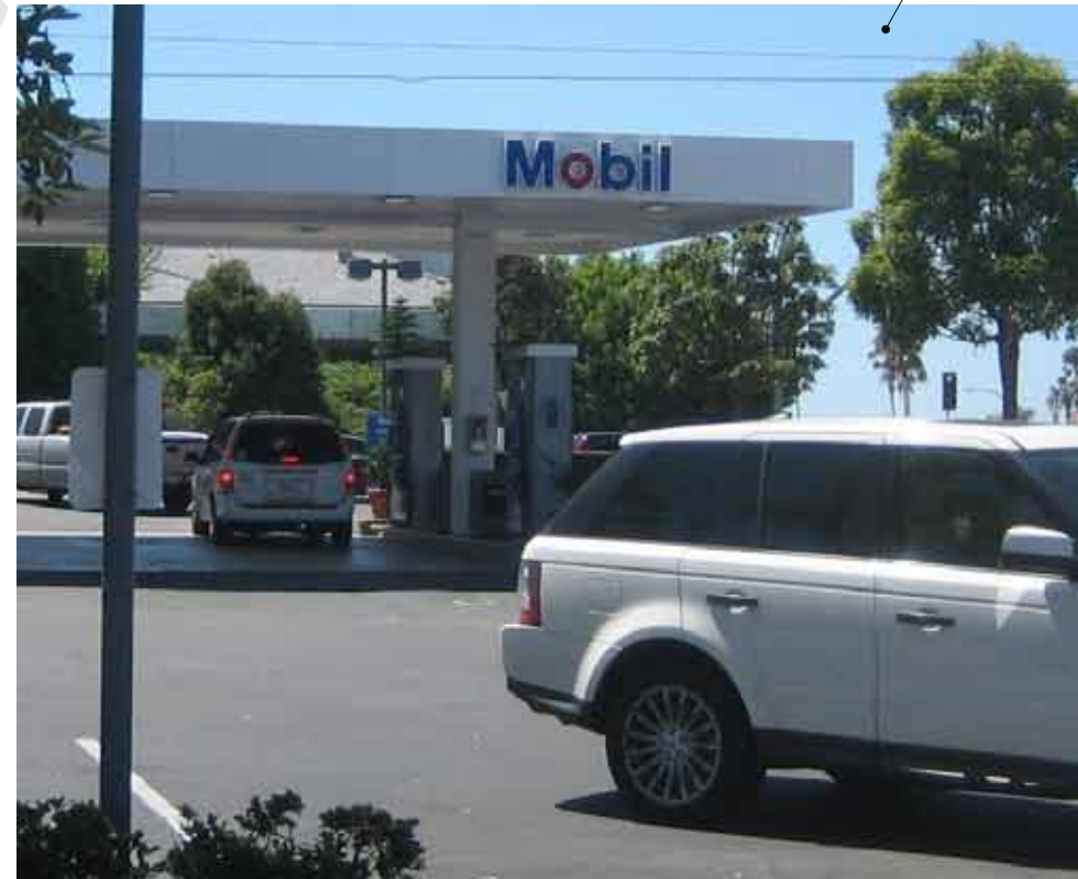
2 EXISTING CONDITION - MOBIL CANOPY SIGN
